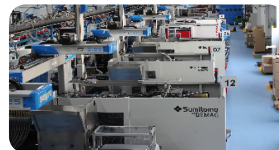
The new injection workshop
